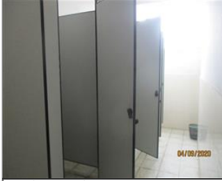
Photo of the sanitary facilities Toilets.JPG
